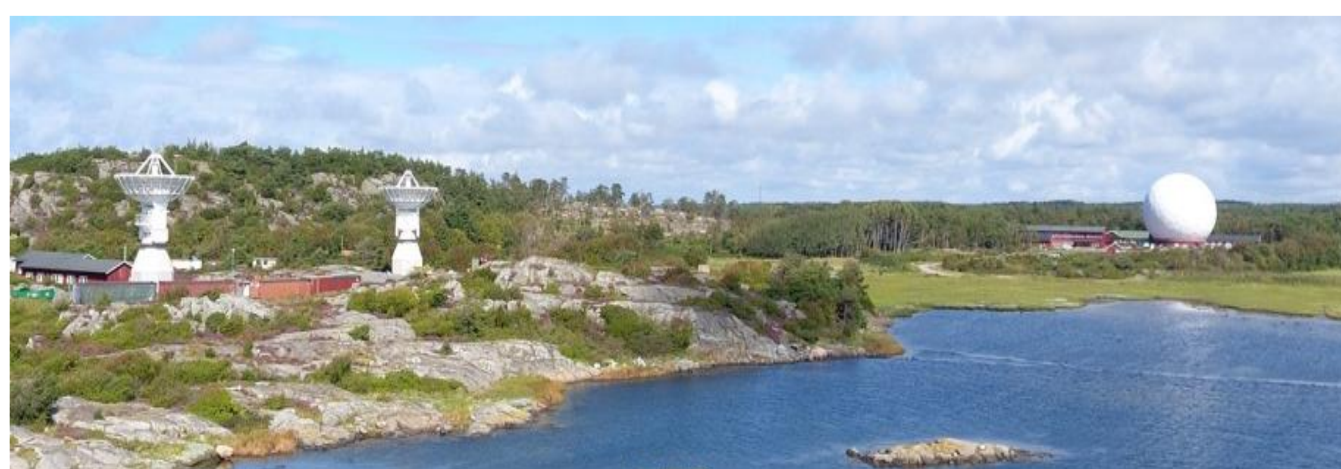
Figure 2: The Onsala twin telescopes and the radome-enclosed Onsala 20-metre telescope, all used for geodetic VLBI.
