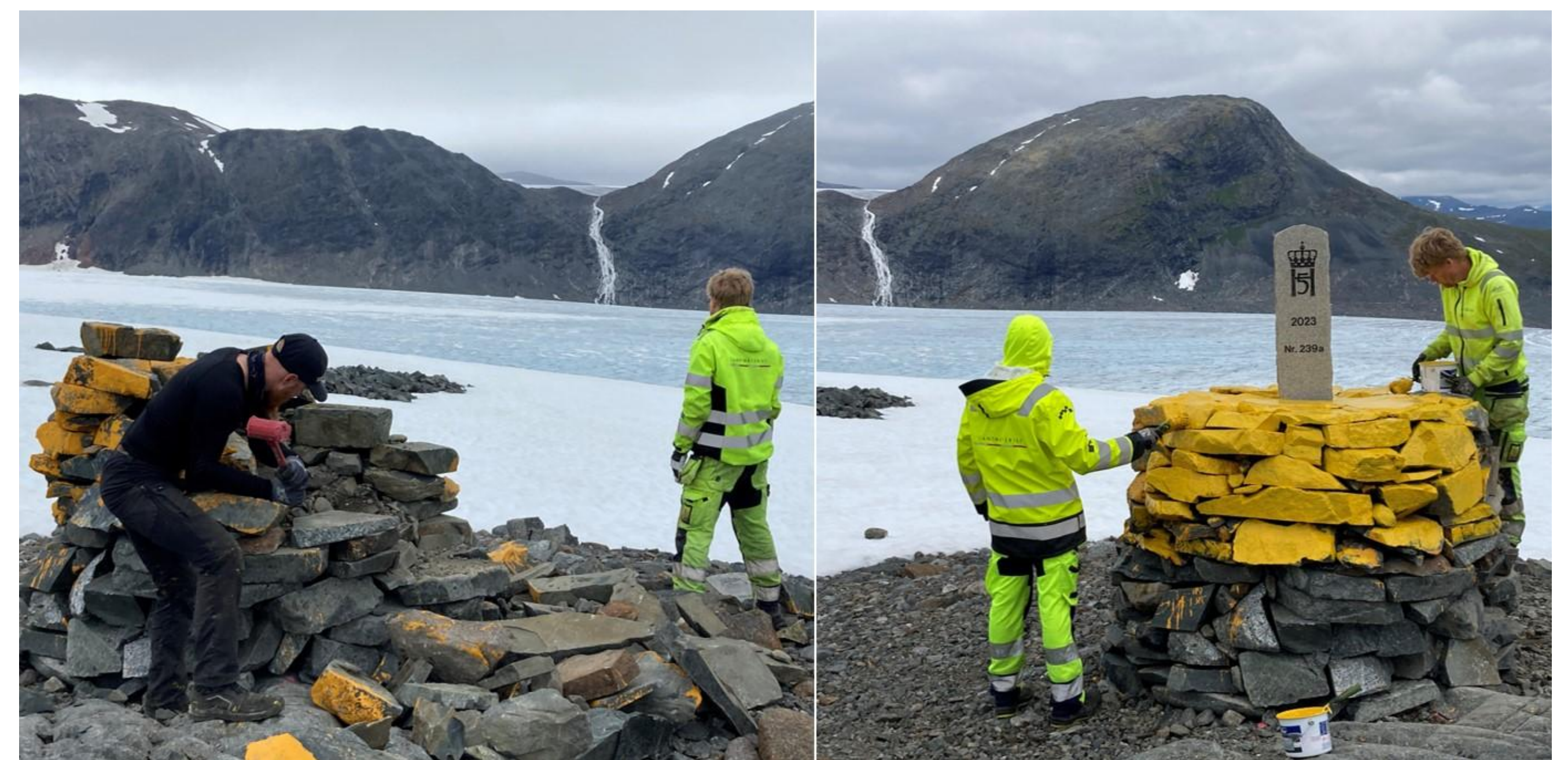
Figure 3: All boundary markers have been thoroughly restored and it have in some places been necessary to replace the central stone with a new one.
