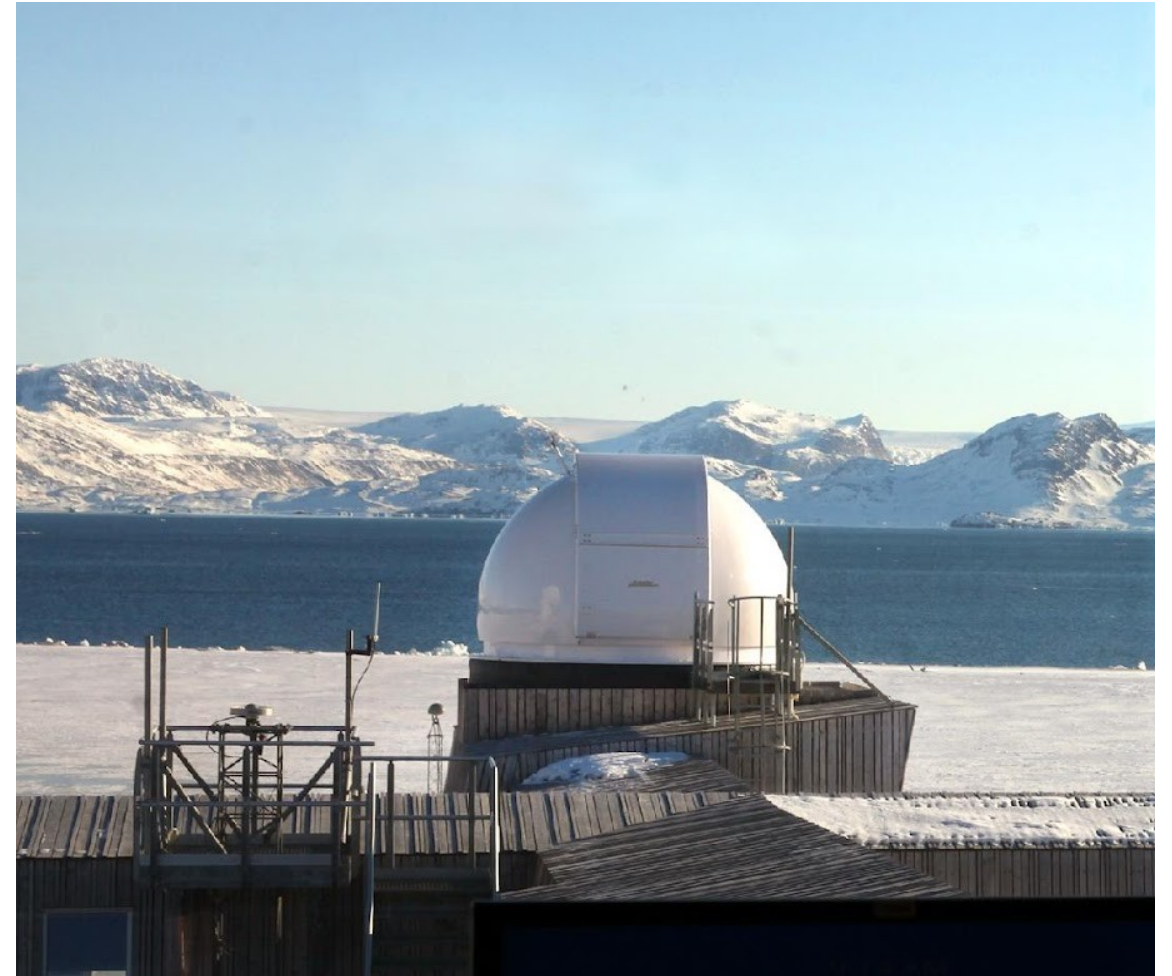
Dome and riser is installed in 2022.
