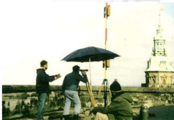
Figure 11: Trigonometric water crossing over Oresund between Kronborg and Pilsjö klint in 1981, using Wild N3, a joint project between KMS and LM.
