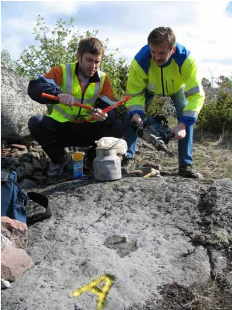
*Figure 4-8. Establishment of an auxiliary marker. (Photograph J. Ahola)*
