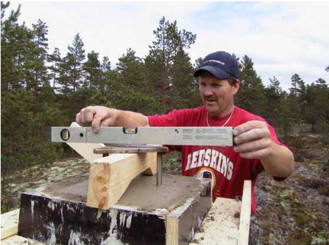
**Figure 4-4.** A proper position of the antenna platform is measured with a builder's level when the pillar was casted. After that the platform cannot be adjusted. (Photograph J. Ahola.)
