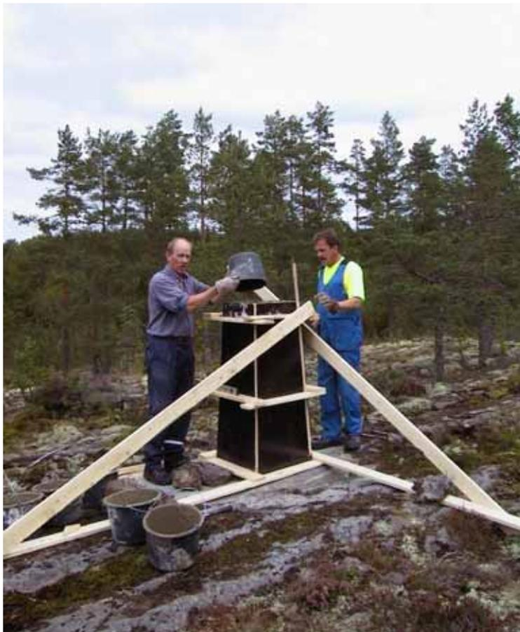
**Figure 4-2.** City of Pori surveyors have been built most of the observation pillars. (Photograph J. Ahola.)
