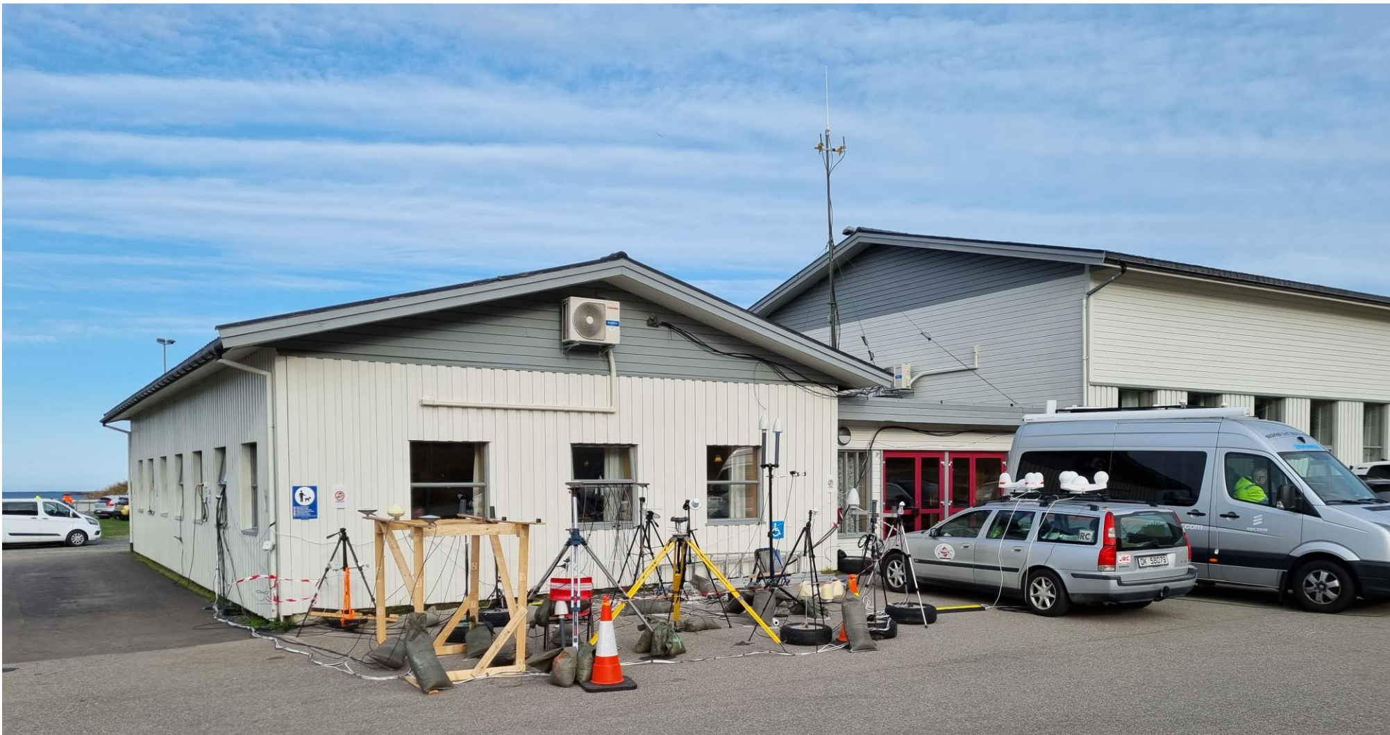
Main GNSS antenna farm outside the house
