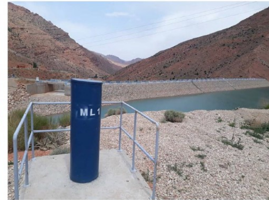
Mojen reservoir rockfill dam
