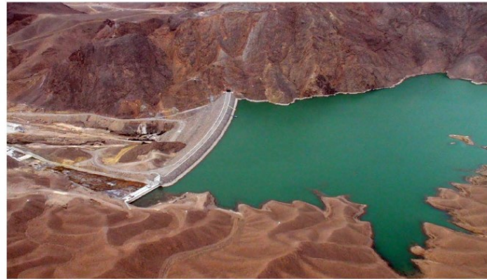
Damghan reservoir rockfill dam
