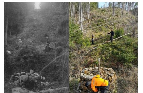
**Figure 4:** The fieldwork during the review of the national boundary 1929–1930 was done in a similar way as during the ongoing review. Rr A close to Idefjorden in the south is however nowadays positioned with more modern surveying technique. Picture: Lars Pettersson.
