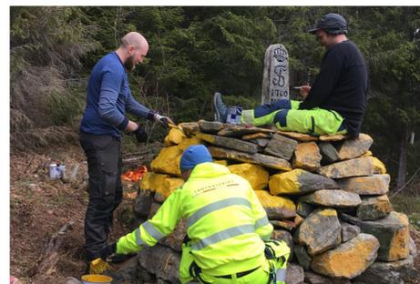
**Figure 3:** During the ongoing review of the national boundary 2020–2024, all boundary markers are restored, painted yellow and measured. The inscriptions on the central stone are filled in with black paint. Picture: Dan Norin.
