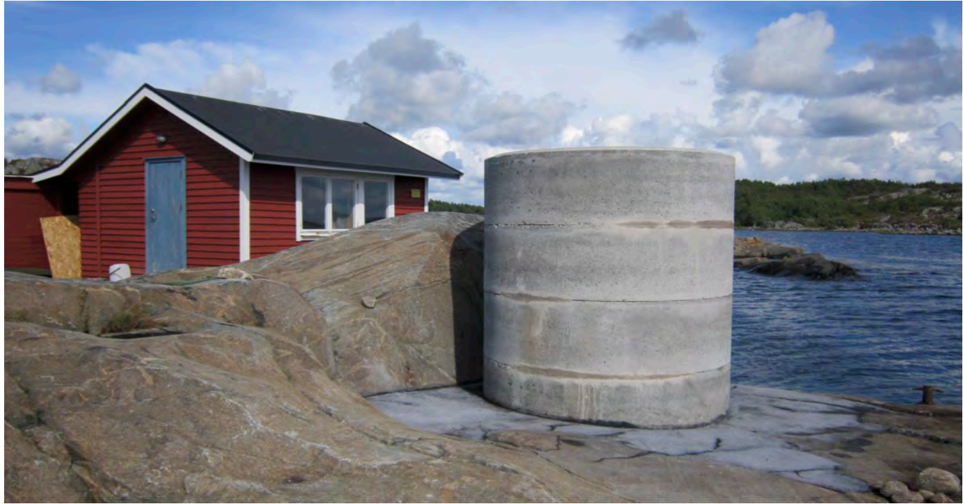
Bubbler and radar sensor tide gauge
