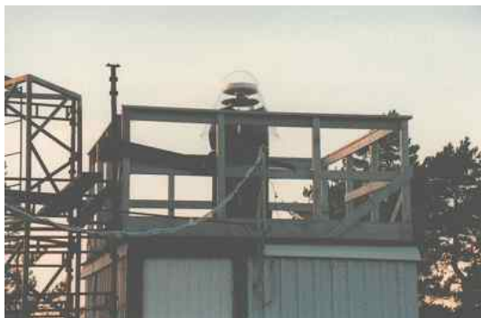
Lovö GPS station: Hut built around pillar with a fence on the roof Steel construction in the south direction
