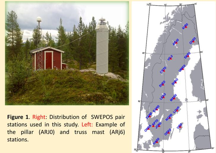
Figure 1. Right: Distribution of SWEPOS pair stations used in this study. Left: Example of the pillar (ARJ0) and truss mast (ARJ6) stations.
